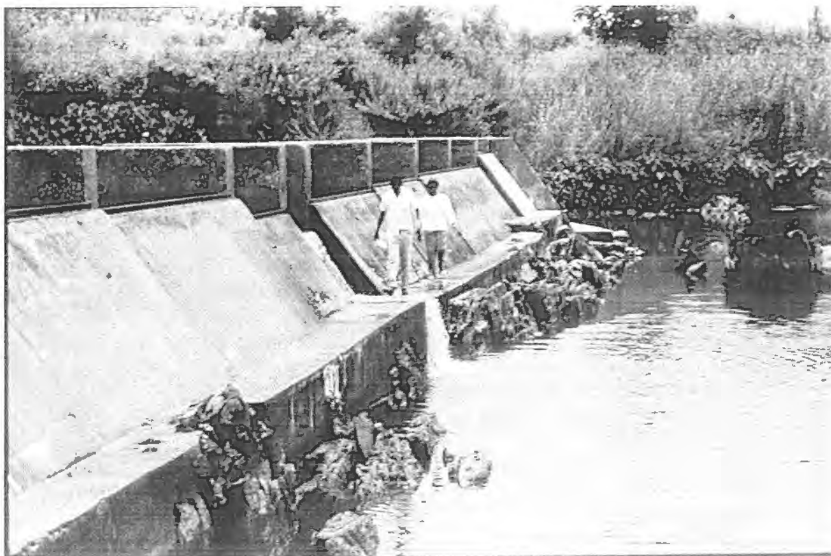
Figure 3.1. The gauging weir at the hydrological station C74.
